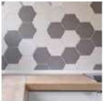
DADO CERAMIC TILES 400 MM ABOVE THE COUNTER
