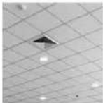
CEILING GRID FALSE CEILING
