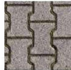
INTERNAL ROADS INTERLOCKING BLOCKS/ TREMIX CONCRETE ROAD
